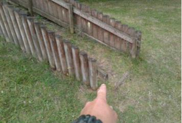
Finding: A barrier support is missing Action: Replace
