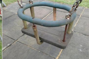
**Finding:** The seat is severely damaged and requires replacing
