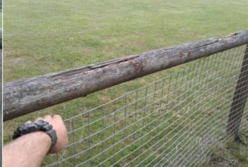
Finding: Sections of mesh are unsecured/ damaged
