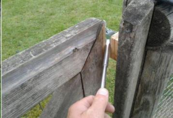
**Action:** Where possible a 12mm gap should be maintained on both sides or between the gate leafs
