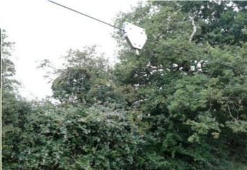
Finding: The suspension and seats was missing at time of Action: Replace as required inspection
