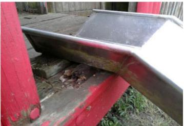
**Finding:** There are areas or parts of the timber on the slide **Action:** Replace all affected timbers starting section that have rotted
