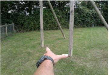
Finding: The timber supports on this item has severe rot
