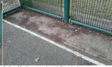
**Finding:** The concrete surface within the goal mouth is damaged
